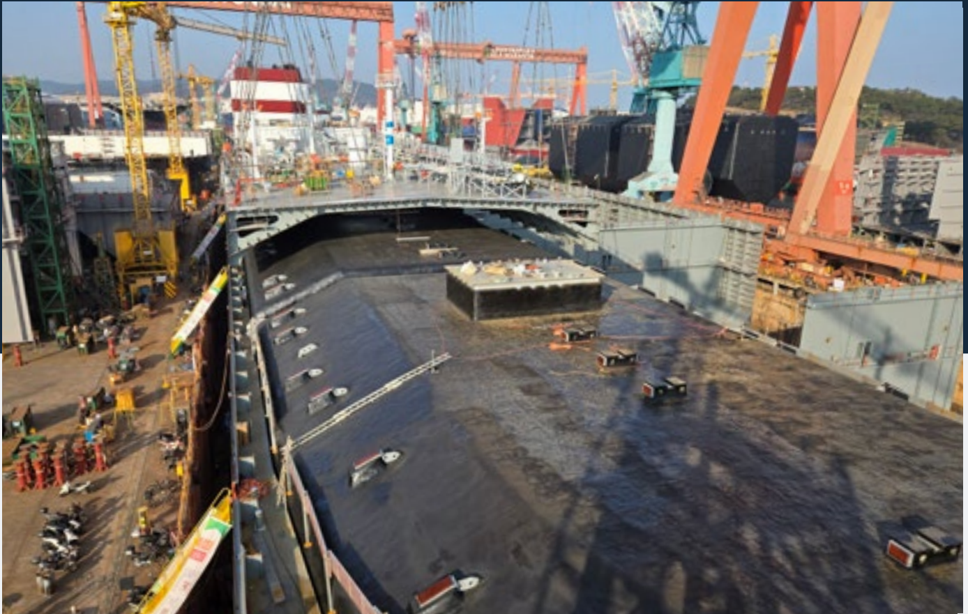
Solvang newbuilding Panamax VLGC under construction in Ulsan, Korea.
